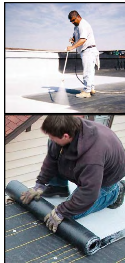
Figure 6: Two Cool Roof Installations
